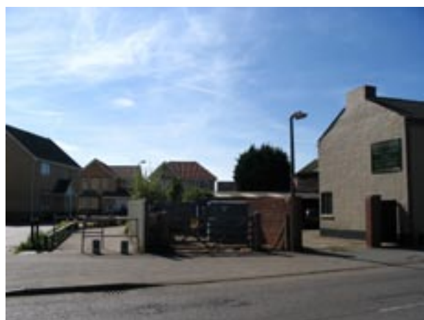
Turnbridge Court & sub-station
