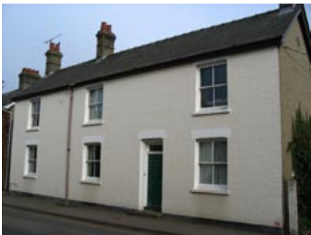
No. 6 & 8 Station Road
