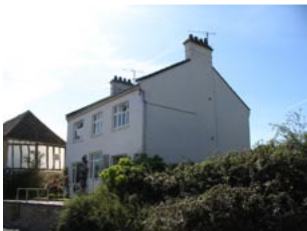
No. 33 Station Road
