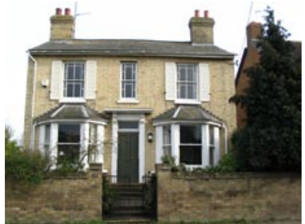
No. 26 Station Road
