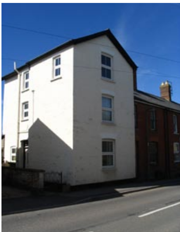
No. 13 Station Road
